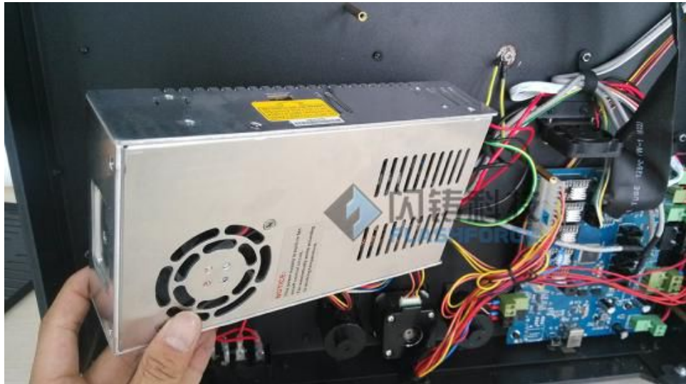
Replace with the new power supply
